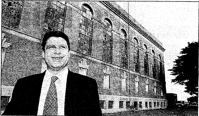
Big project: Steve Bracks wants to see as many Hobsons Bay residents as possible at the old substation next week.
