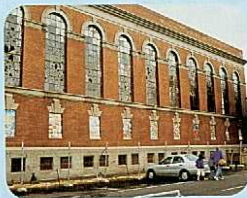
The Newport Sub Station in its current state.
